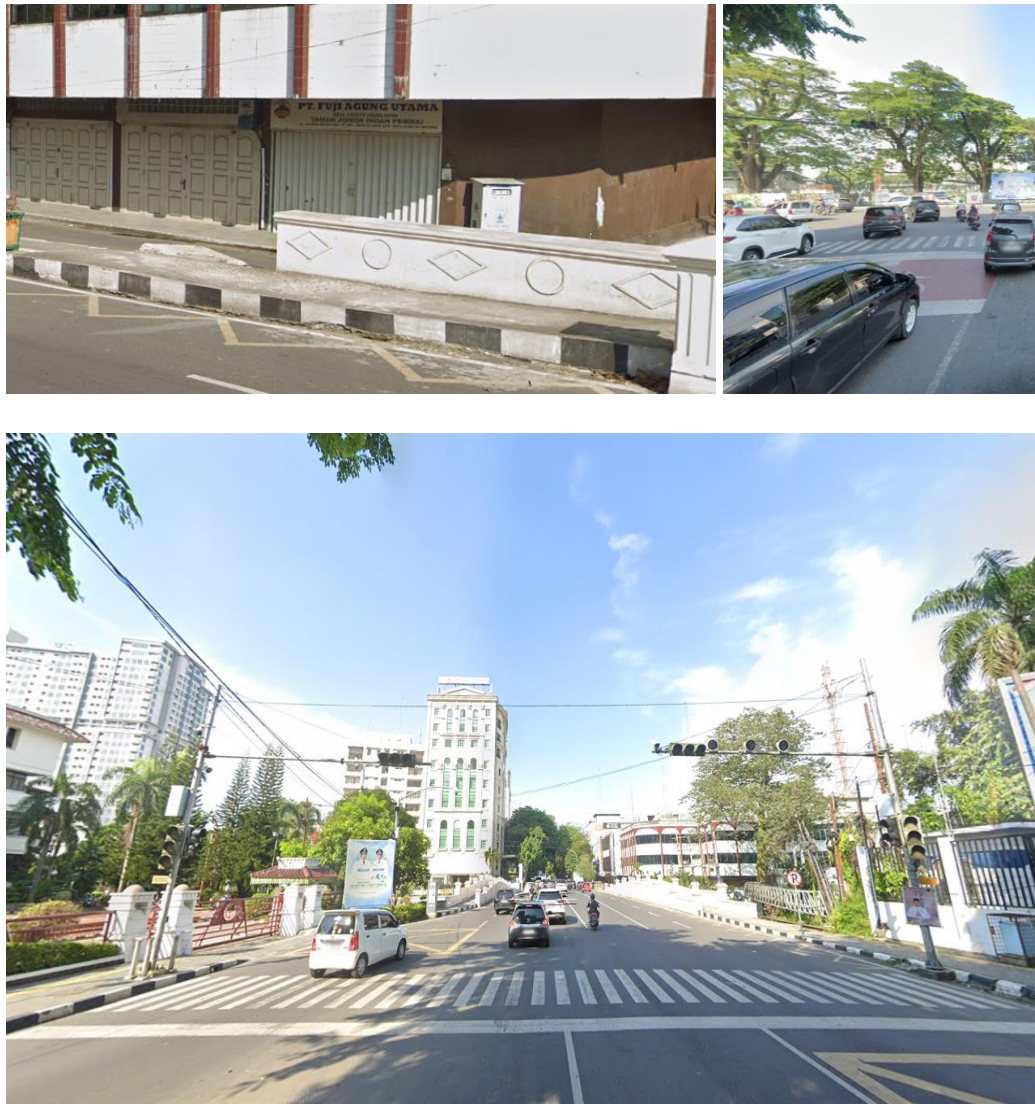
Figure 3. Pedestrian conditions are characterized by narrow, damaged sidewalks and hazardous crossing points."
