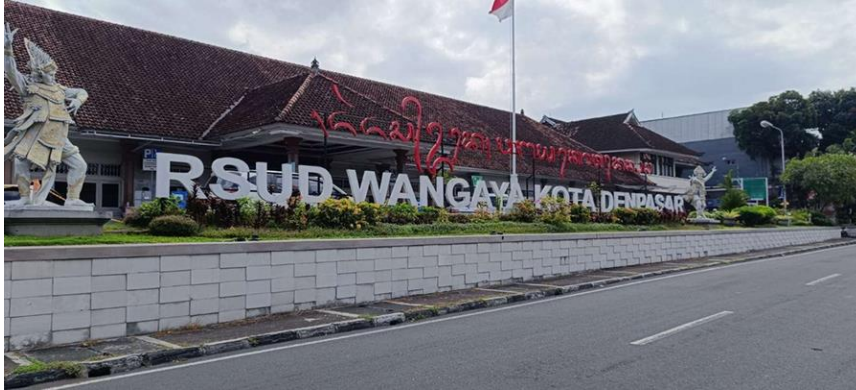
Figure 1. Front View of Wangaya Hospital Denpasar City Source: Personal Documents, 2025
